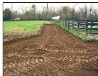
Figure 2. Excavation through the topsoil to stable soil beneath.
