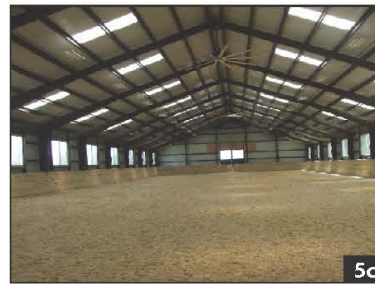
Figure 5. Ventilating through a roof peak (a); large end wall openings for ventilation (b); and side wall windows for ventilation and high-volume low-speed fan for air movement (c)
