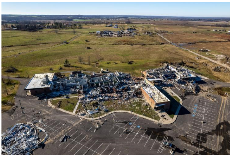
AERIAL VIEW OF THE UK RESEARCH AND EDUCATION CENTER AFTER IT TOOK A DIRECT HIT FROM A WEEKEND TORNADO. PHOTO BY MATT BARTON, UK AGRICULTURAL COMMUNICATIONS.
